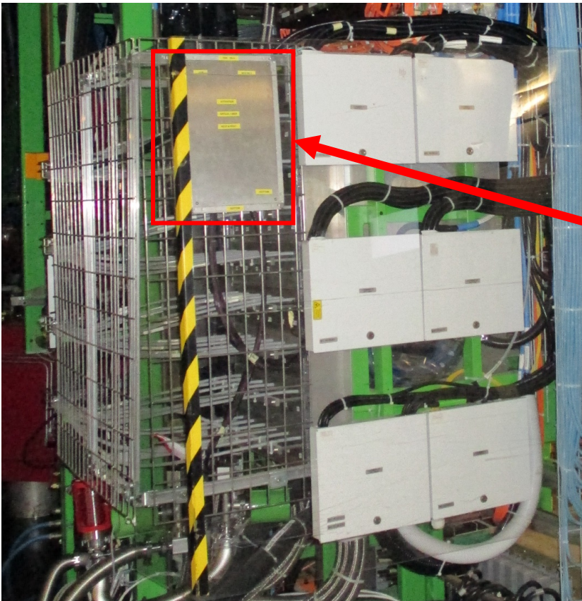
YE+1 Patch pannel RPC Optical Fiber Box
