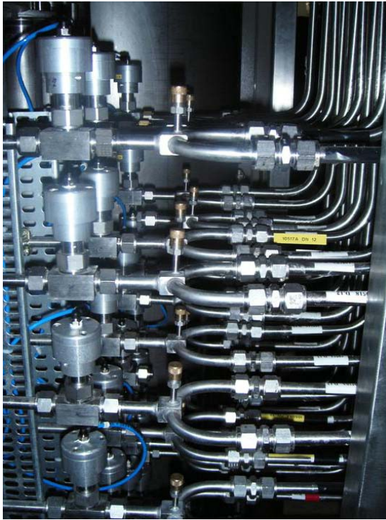
Fig. 6.2.9 – Return manifold
