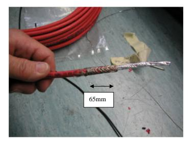
Remove the flame shield from the inner conductors using small sharp snips. Do not damage the insulation on these wires.
