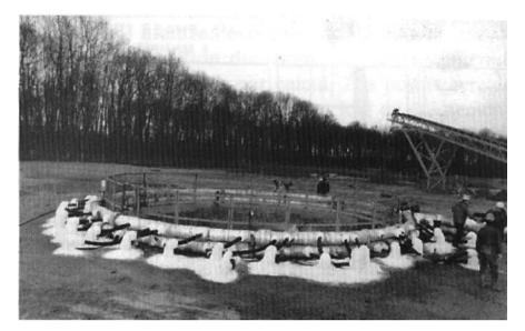
Fig. 4.11 Upper part of a shaft with cryogenic equipment to freeze the ground
