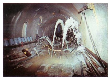
Fig. 4.14 The tunnel flooded by water under the Jura Mountains
