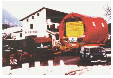
Fig. 7.7 The largest superconducting solenoid ever produced and destined for DELPHI had to be transported to CERN on roads without bridges but difficulties were still encountered in narrow passages
