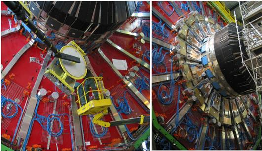
Figure 9. Installation of the very first CSC+RE1/2 module (left); 36 RE1/2s for one endcap have been installed on CMS before December 2005 (right).
