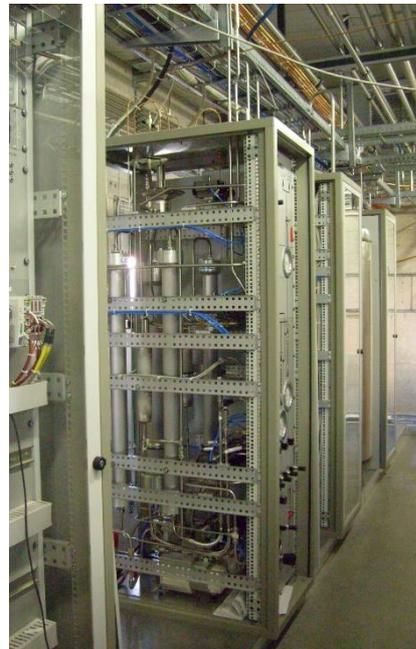
*Fig. 4.1.2 Overview of the CF<sub>4</sub> recuperation plant installed in the surface gas building (SGX5) of the CMS experiment.*
