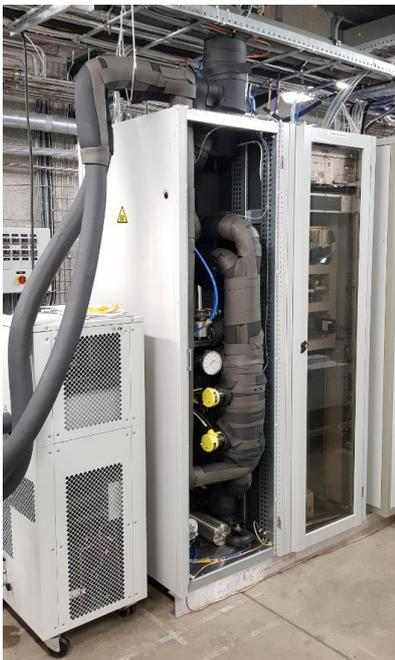
*Fig. 4.1.1 First prototype of the R134a recuperation plant successfully tested recently at CERN in the RPC detector system.*
