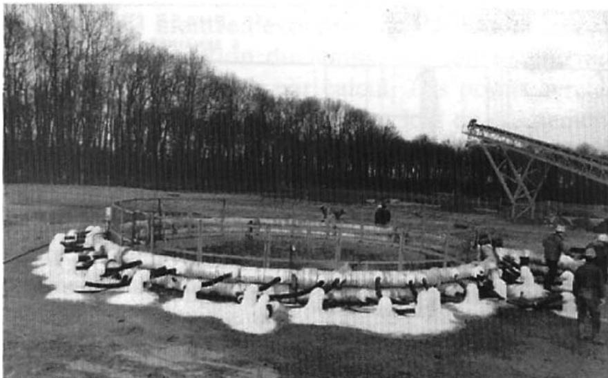
**Fig. 4.11** Upper part of a shaft with cryogenic equipment to freeze the ground
