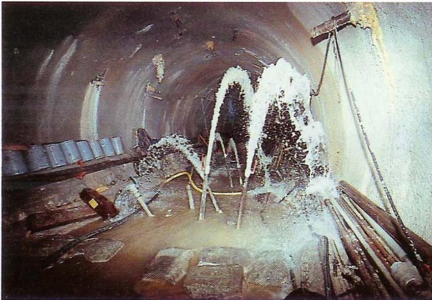
Fig. 4.14 The tunnel flooded by water under the Jura Mountains
