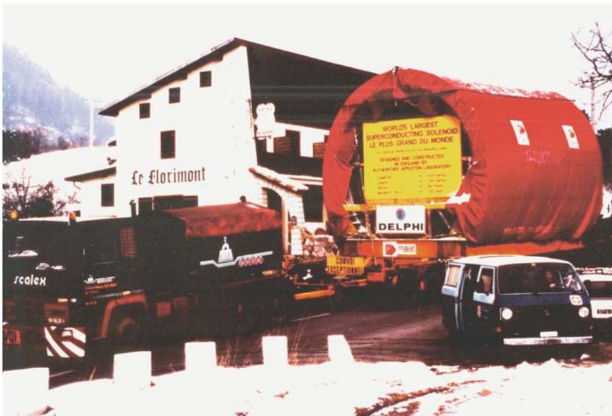
**Fig. 7.7** The largest superconducting solenoid ever produced and destined for DELPHI had to be transported to CERN on roads without bridges but difficulties were still encountered in narrow passages
