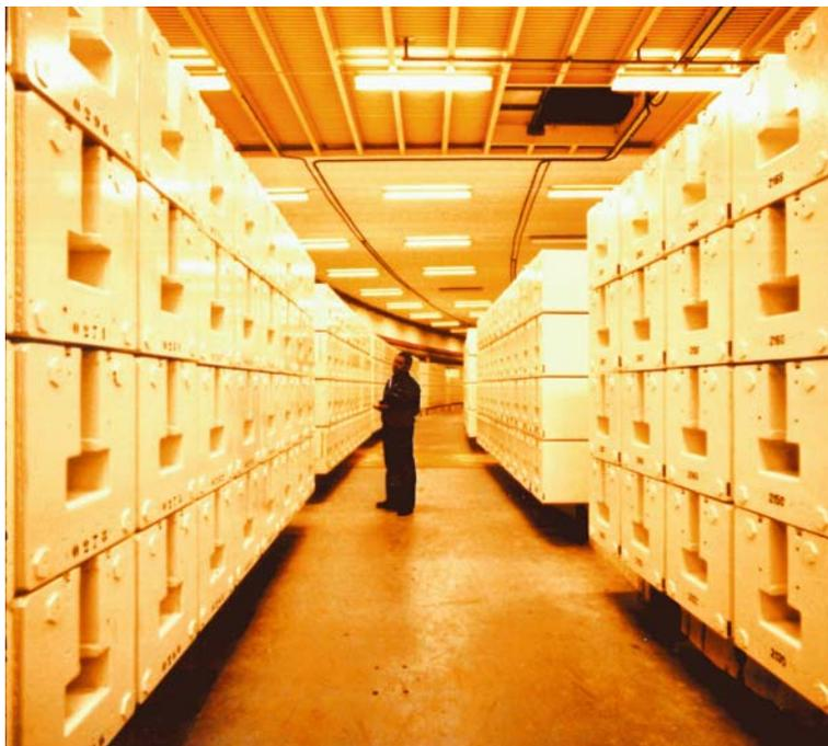
**Fig. 6.4** The storage of the bending magnets in the old Intersecting Storage Rings (ISR) tunnel
