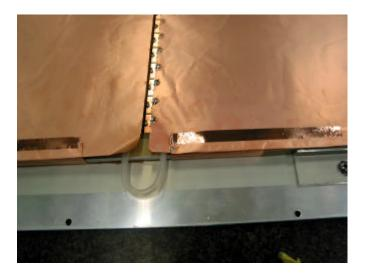
Solder on the signal reference cable that has been identified as such, using letters (Scem.....). Use cable 'x' mm<sup>2</sup> (Scem.....)
